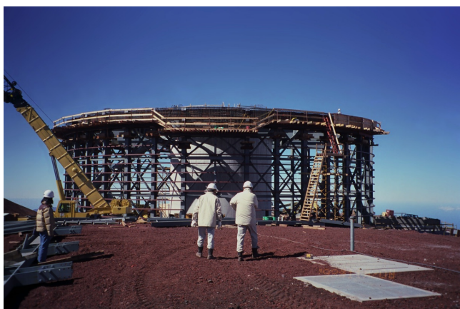
The iron structure of the lower (fixed) part of the enclosure building with the concrete-pier of the telescope at its center.
