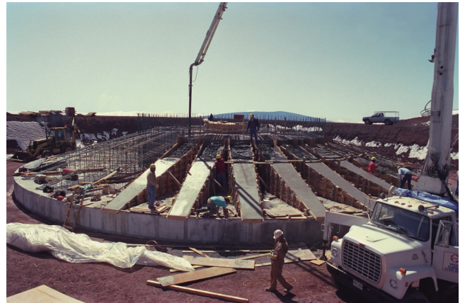
The bottom part of the concrete pier is made. ©NAOJ
