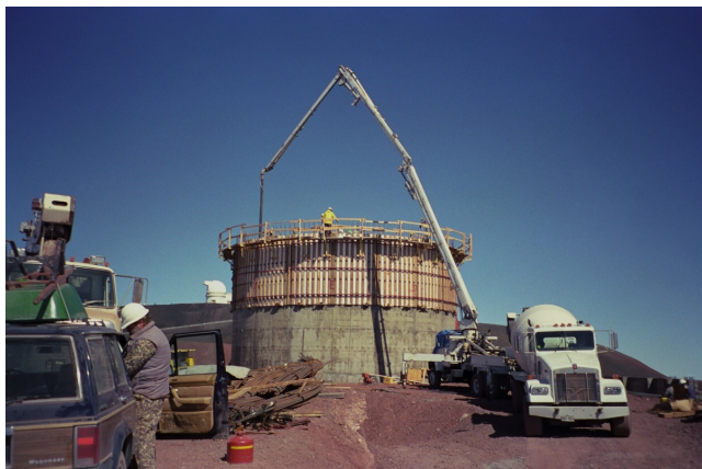
Concrete pier is now half-way. ©NAOJ
