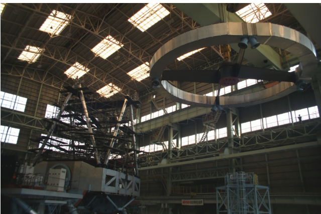
The top ring is lifted up. It will be moved to the left and will be put on the Cerrurier Truss structure.
